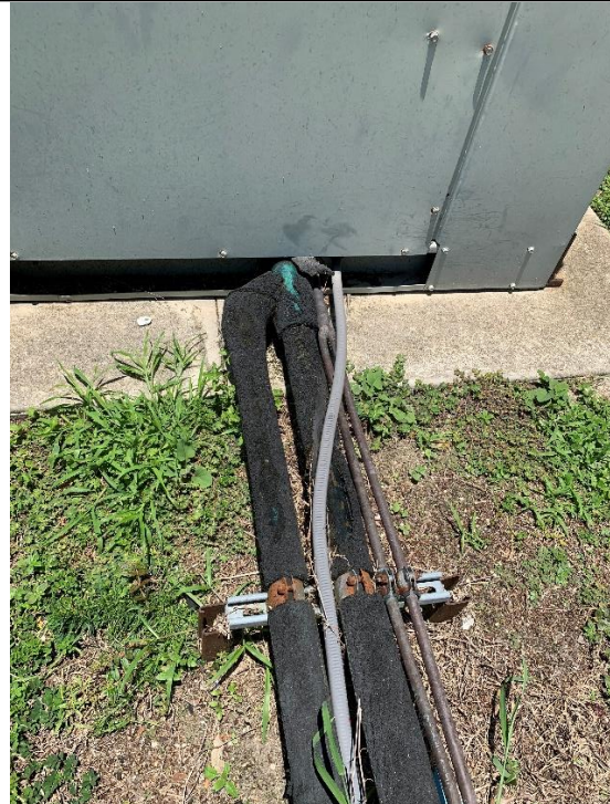
Figure 4 – Liquid Line out from CU-2
