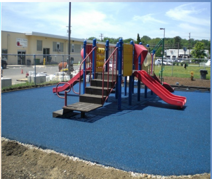
Rolled Edge for Surrounding Loose Fill
