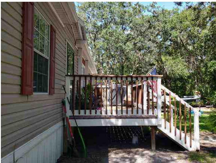
Additional view of front wood deck
