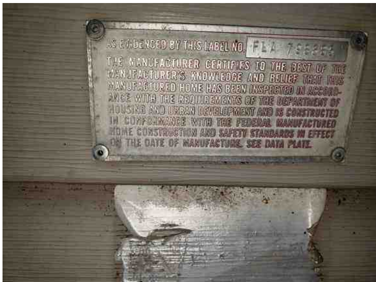
HUD label FLA 798685 located on Rear of home
