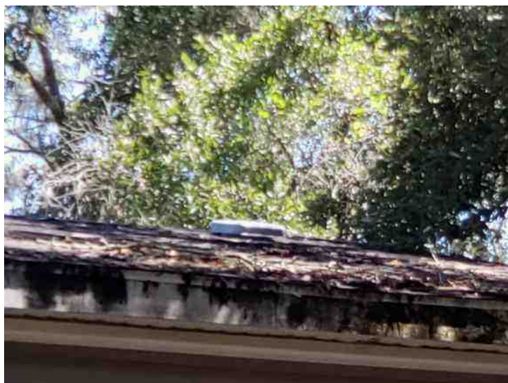
Additional view of roof under trees
