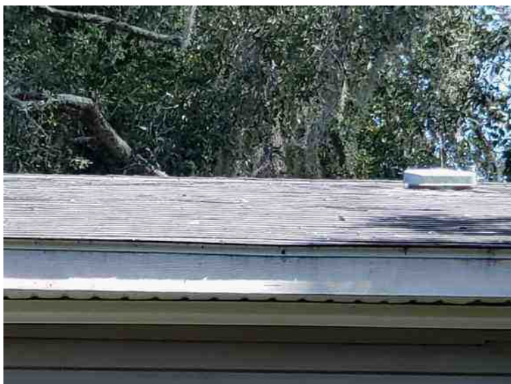
View of roof
