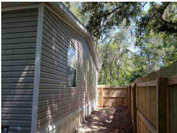
North side of home
