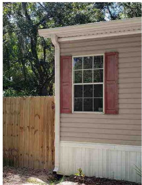
Downspouts and gutters in place
