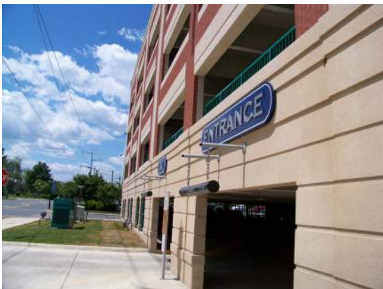
City of Manassas, Manassa, VA Signage Designed By KMA Design
