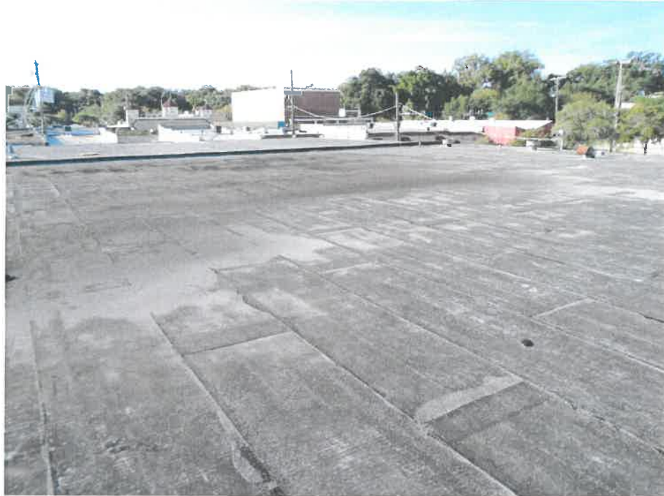
Figure 3: North section of the roof looking south.
