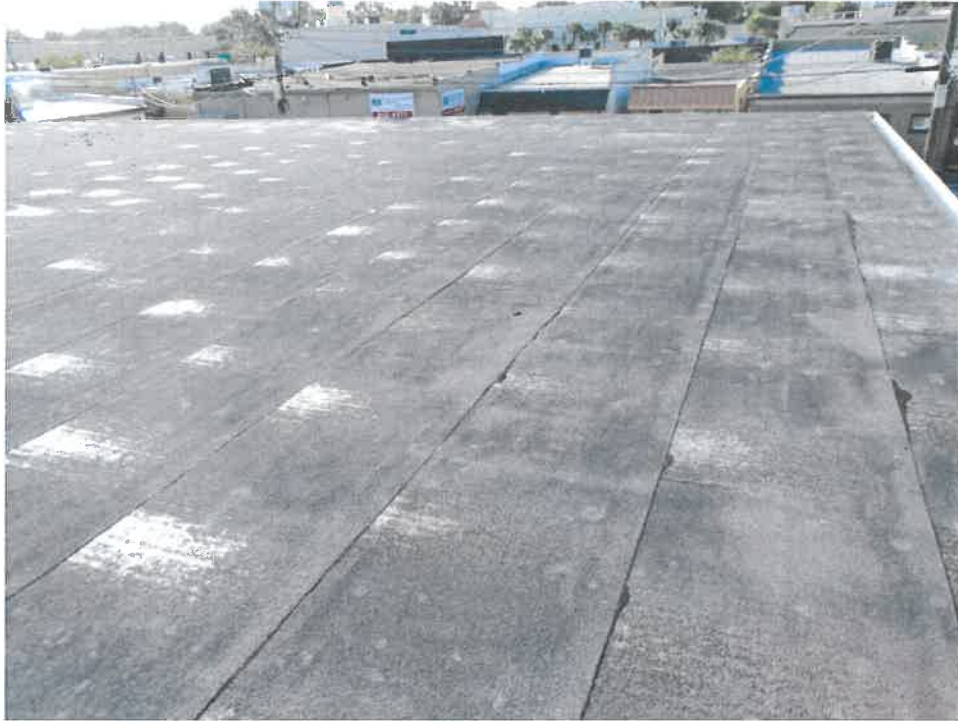
Figure 11: The south section of roof looking south.
