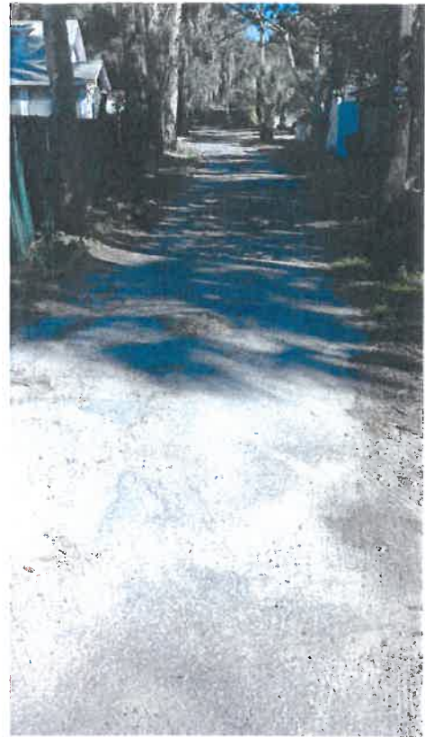
Figure 2 - Typical roadway grade 2 (Queens Ln.)
