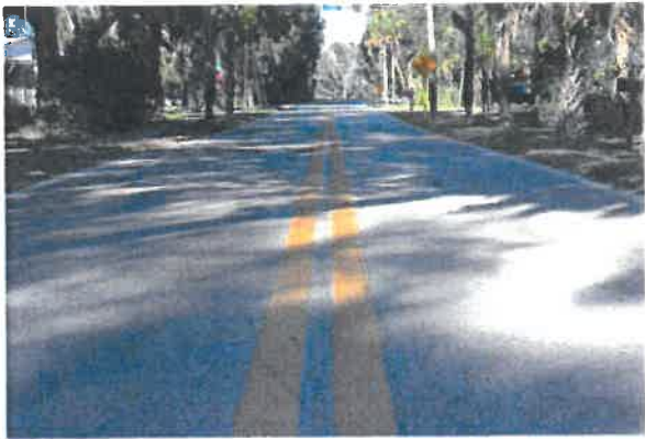
Figure 1 - Typical Roadway Grade 8 (Grand Blvd.)
