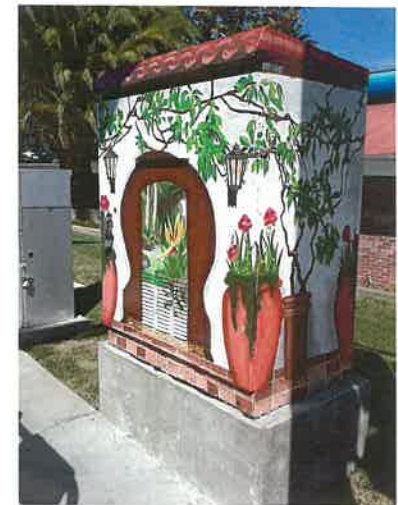
Painted Signal Box
