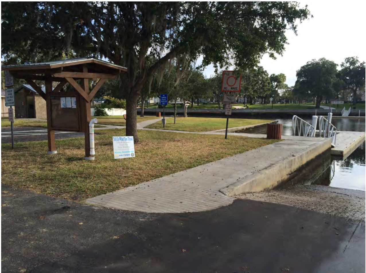
Figure 1.10 – Sims Boat Ramp – Example of a Special Purpose Facility
