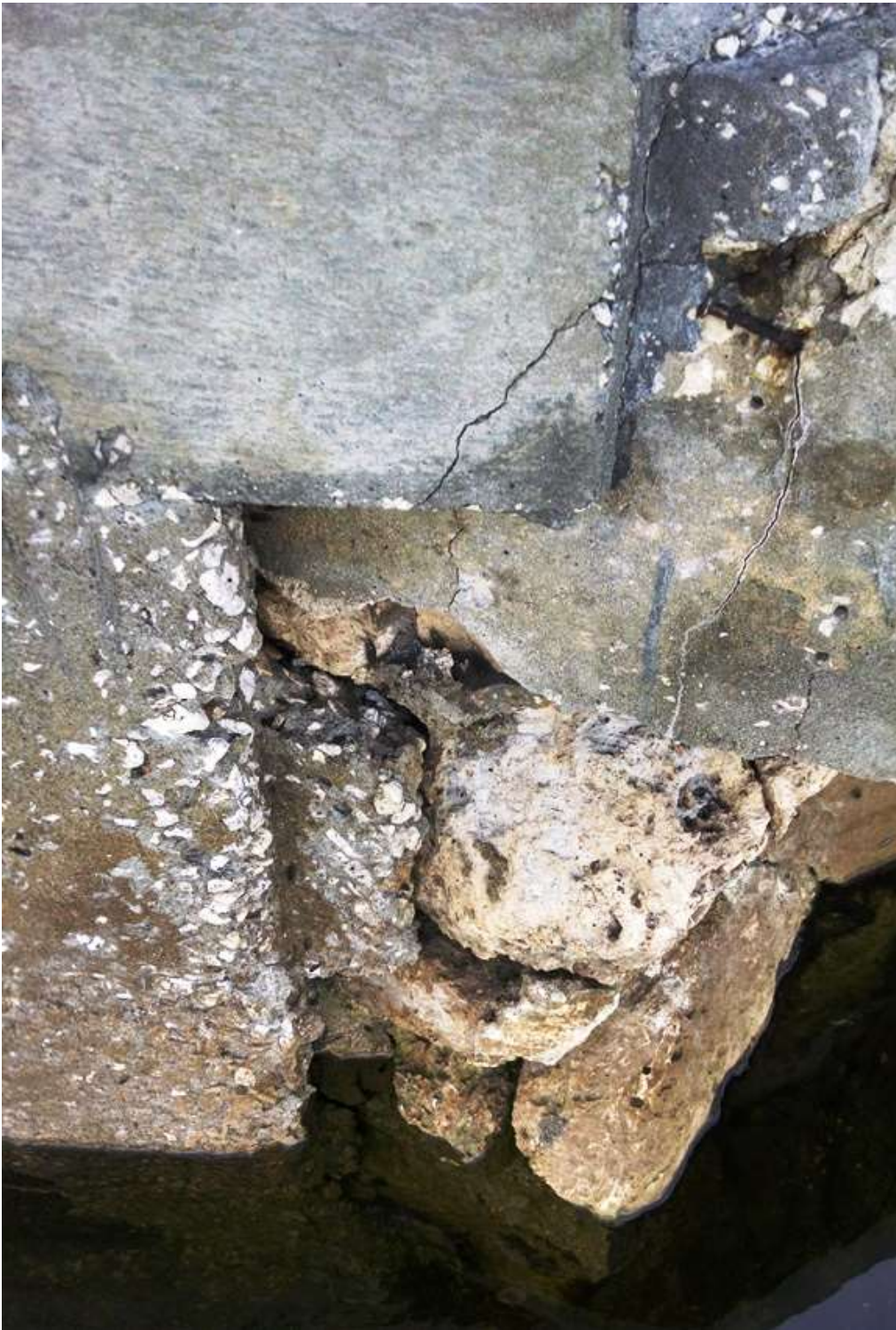
Figure 12 – Wall Crack/Spalling
