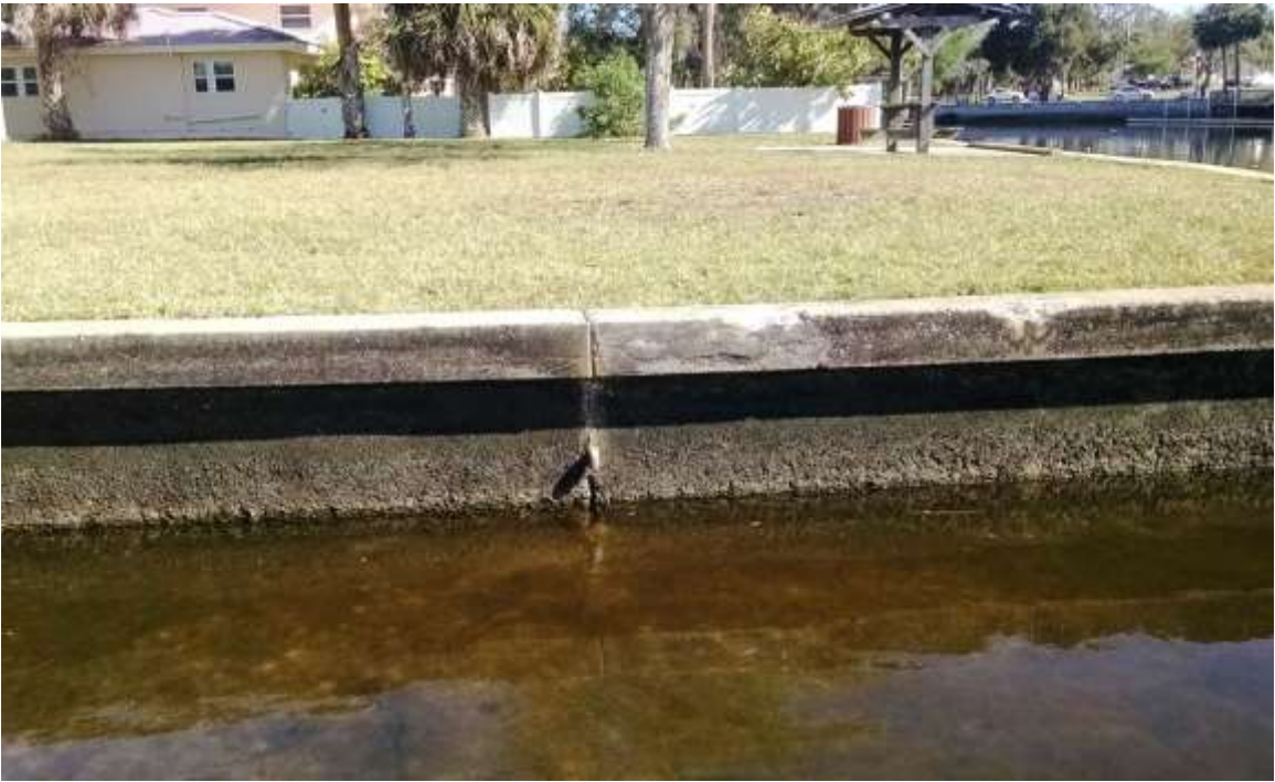
Figure 6 - Drainage Pipe at Wall Joint
