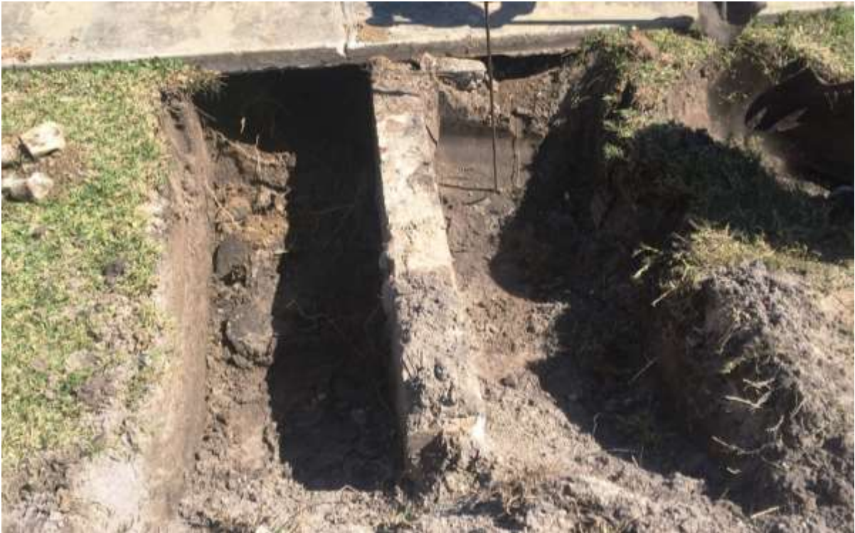
Figure 26 - Jasmine Park Bulkhead Concrete Tie-Back Excavation
