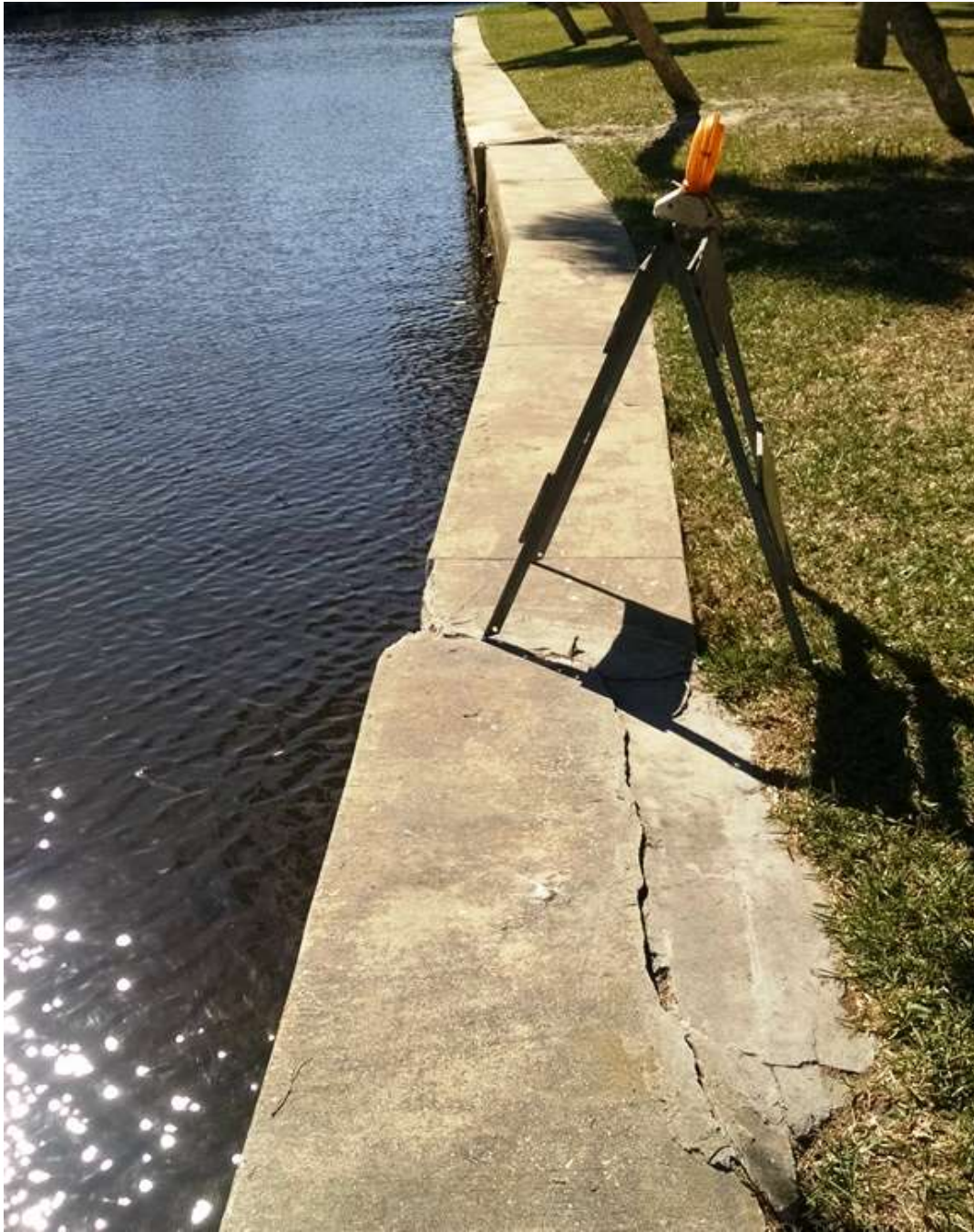
Figure 22 - Wall Failure/Crack
