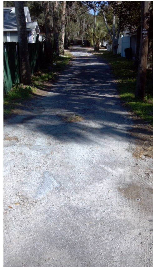
Figure 2 - Typical roadway grade 2 (Queens Ln.)
