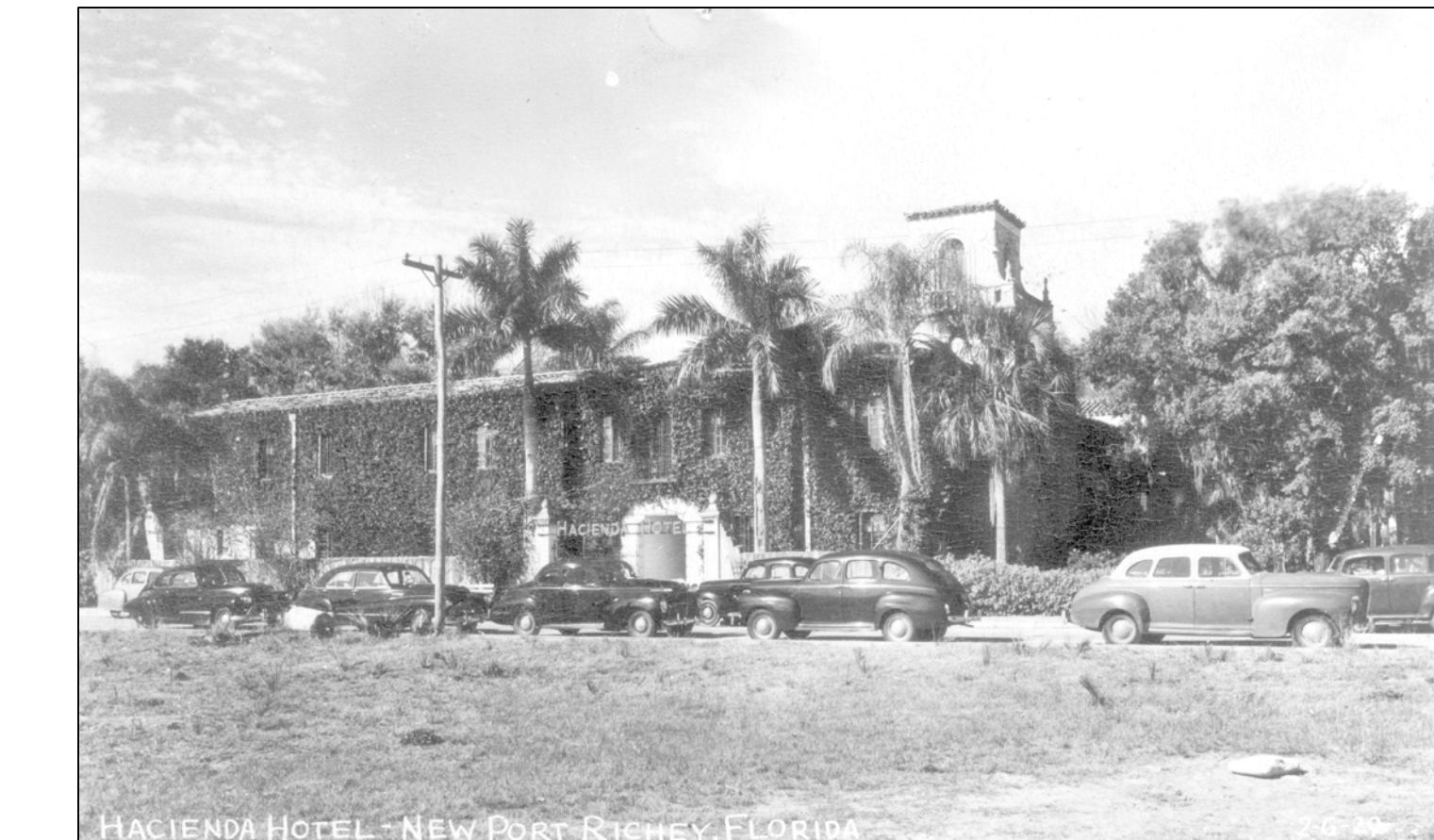
4 EAST FACADE OF BUILDING, 1940'S PHOTO A8.0 SCALE: N.T.S.
