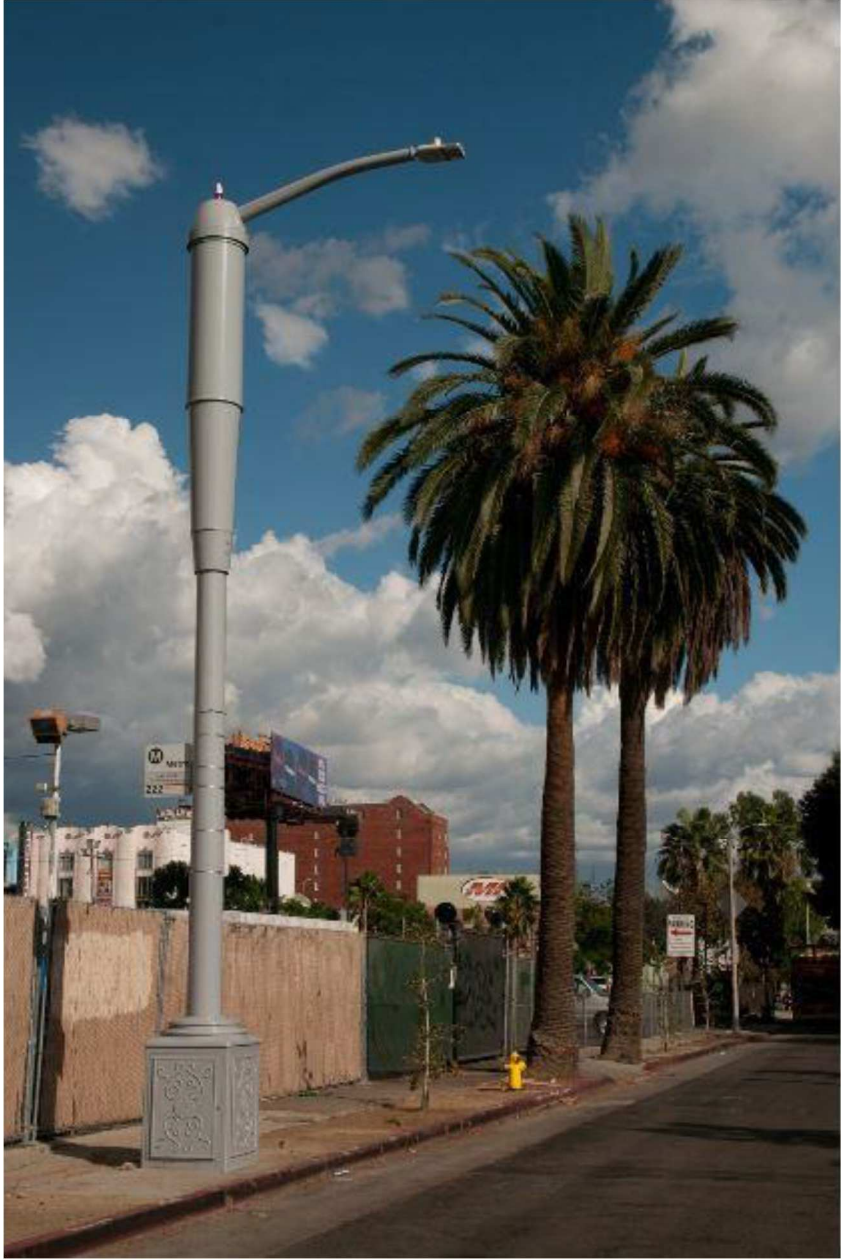
Exhibit 5. The antenna enclosure has a larger diameter than the pole, rendering it insufficiently cloaked. This design is prohibited.
