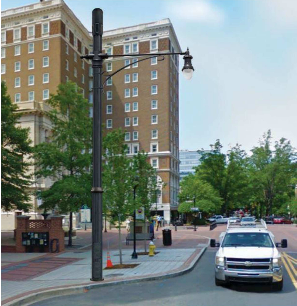
Exhibit 1. Example of a fluted pole with collocated wireless antennas. Actual application should match City of New Port Richey Light Pole Standards.
