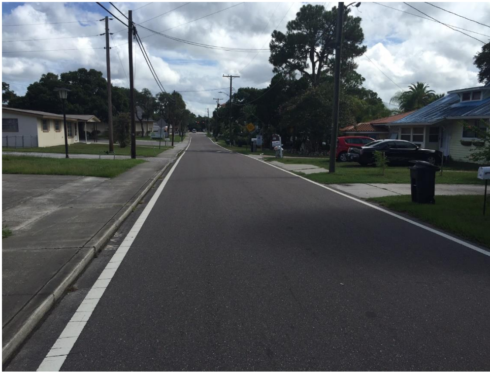
River Road looking north
