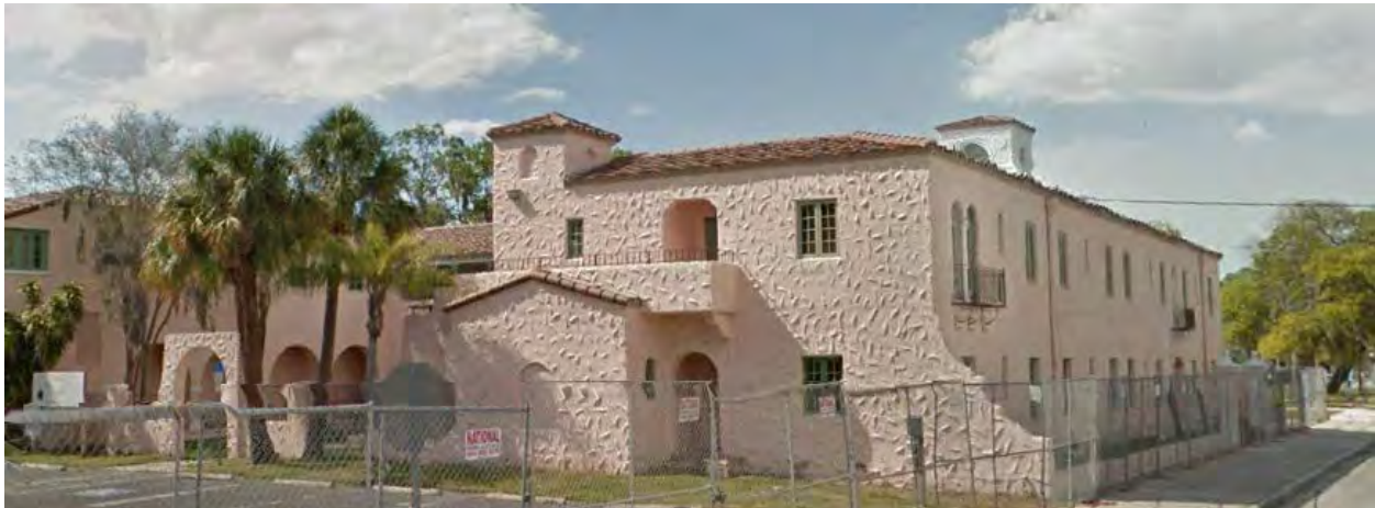
Figure 14: Hacienda Hotel (southeast corner)
