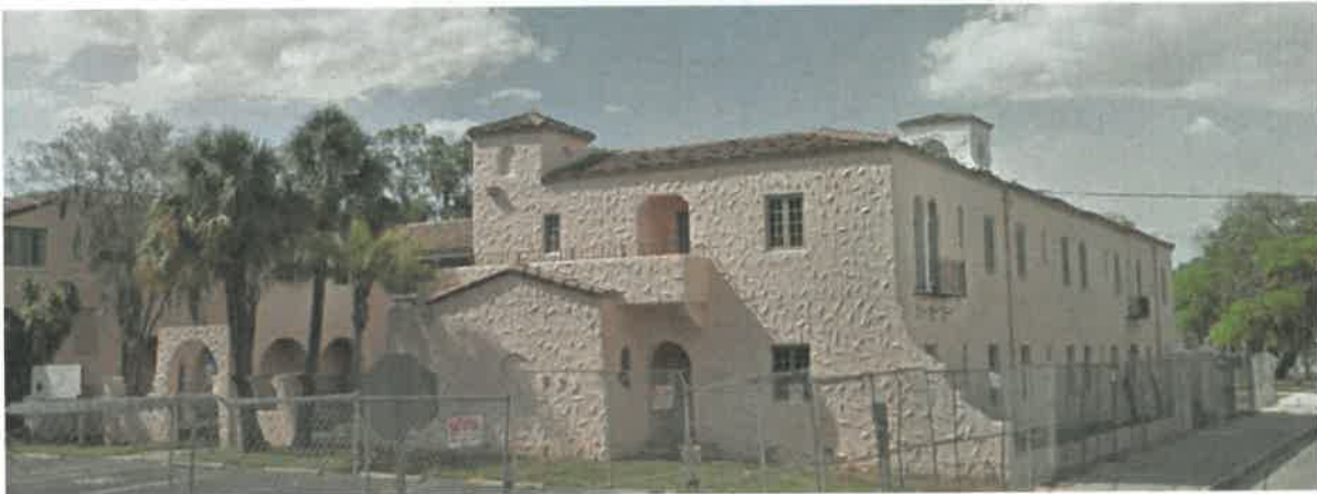
Figure 14: Hacienda Hotel (southeast corner)
