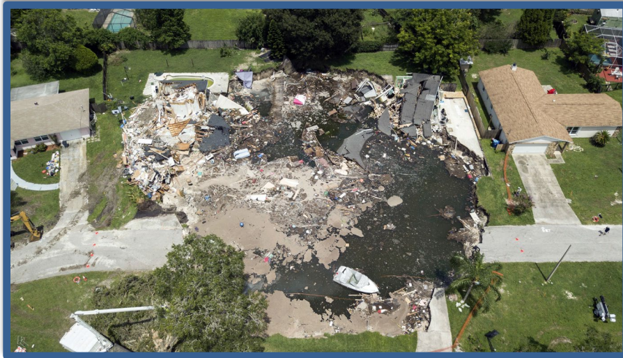
Figure 2.42 July 2017 Land O'Lakes Sinkhole
