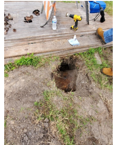
Figure 3-2: Exterior Pipe Corrosion.
