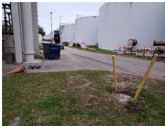
Figure 1-1: City of New Port Richey Water Reclamation Facility
