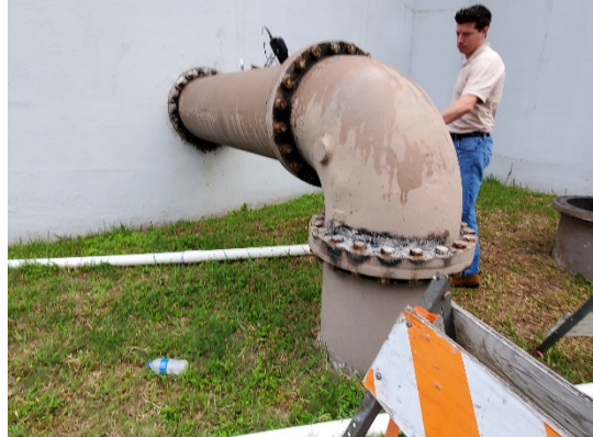
Figure 4-3: Pipe Condition Assessment Field Testing.
