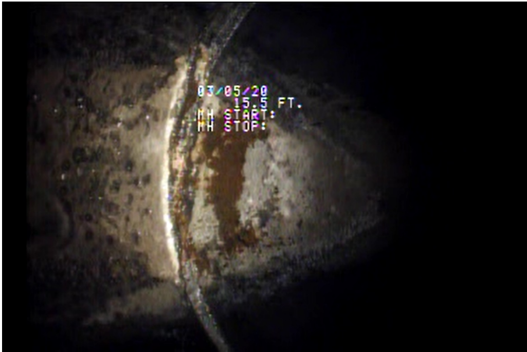
Figure B-4: Pipe Interior at Joints.
