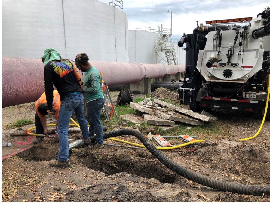
Figure C-9: Vacuum Uncovering of Schreiber Plant Below-Grade Piping (UTT-8)
