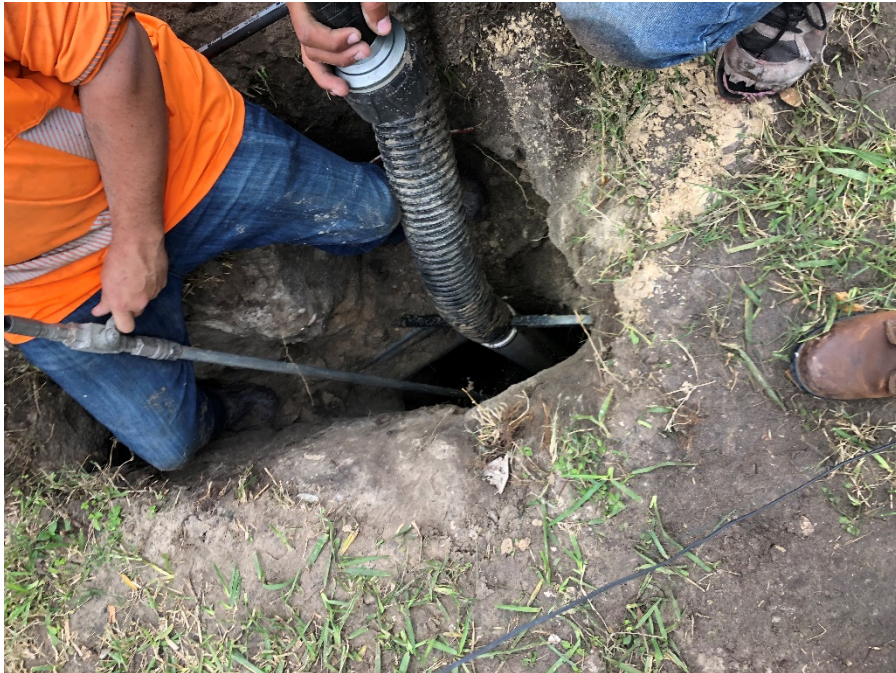
Figure C-12: Vacuum Uncovering of Schreiber Plant Below-Grade Piping (UTT-10)
