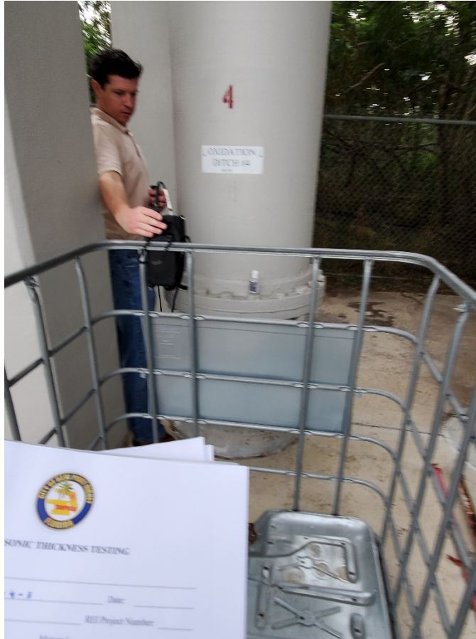
Figure C-5: Oxidation Ditch #4 Headworks Facility Piping (UTT-5)
