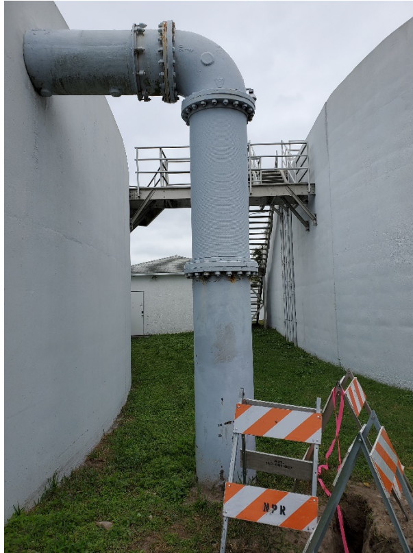
Figure C-7: Schreiber Plant Above-Grade Piping (UTT-7)
