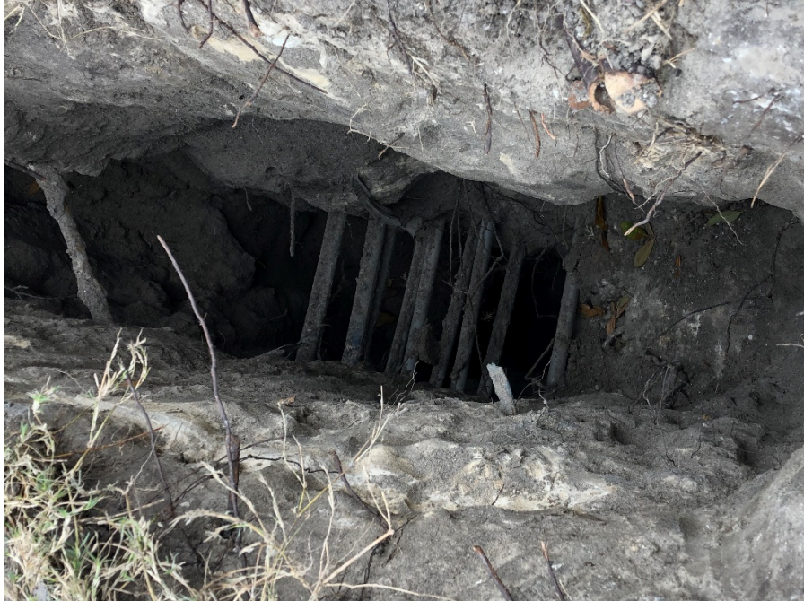
Figure C-11: Schreiber Plant Below-Grade Piping and Crossing Utilities (UTT-9)
