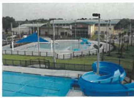
New Port Richey Recreation Center New Port Richey, FL Size: 35,000 Value: $12.7 million
