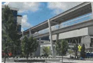
SWA Waste to Energy Skybridge
