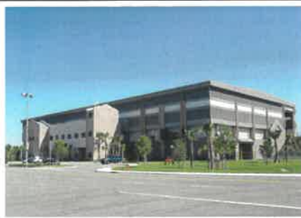
Southwest County Transfer Station Construction - Palm Beach, FL Size: 45,000-sf Value: $26.6 million
