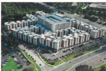
ACC UCF Parking Garage
