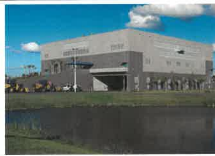
South County Transfer Station Expansion Gibsonton, FL Size: 68,000-sf Value: $19.3 million
