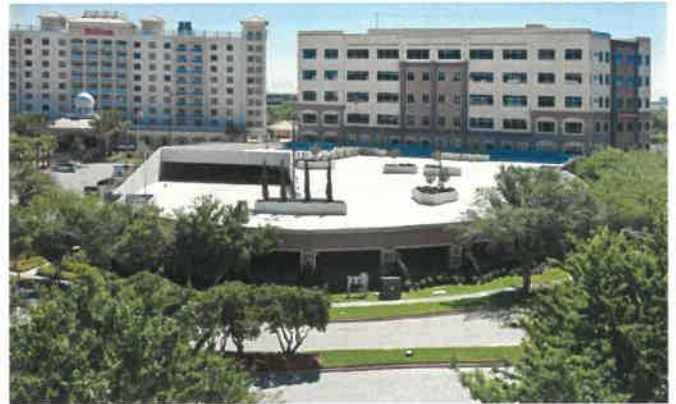
Echelon Pointe at Carillon Parking Garage - St. Petersburg, Florida
