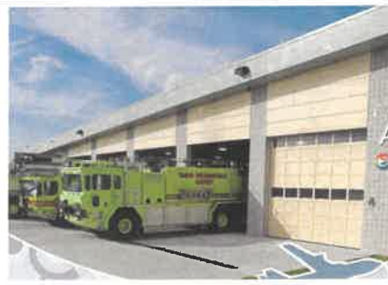
Airport Rescue and Firefighting Facility Tampa International Airport, FL Size: 27,500-sf Value: $5 million
