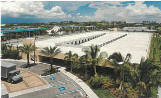
Cypress Bay Executive Center Parking Garage - Tampa, Florida
