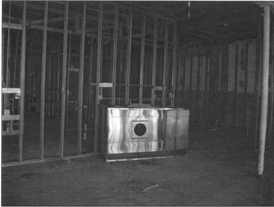
INTERIOR VIEW 2 ND FLOOR
