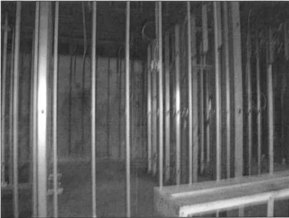
INTERIOR VIEW 2 ND FLOOR
