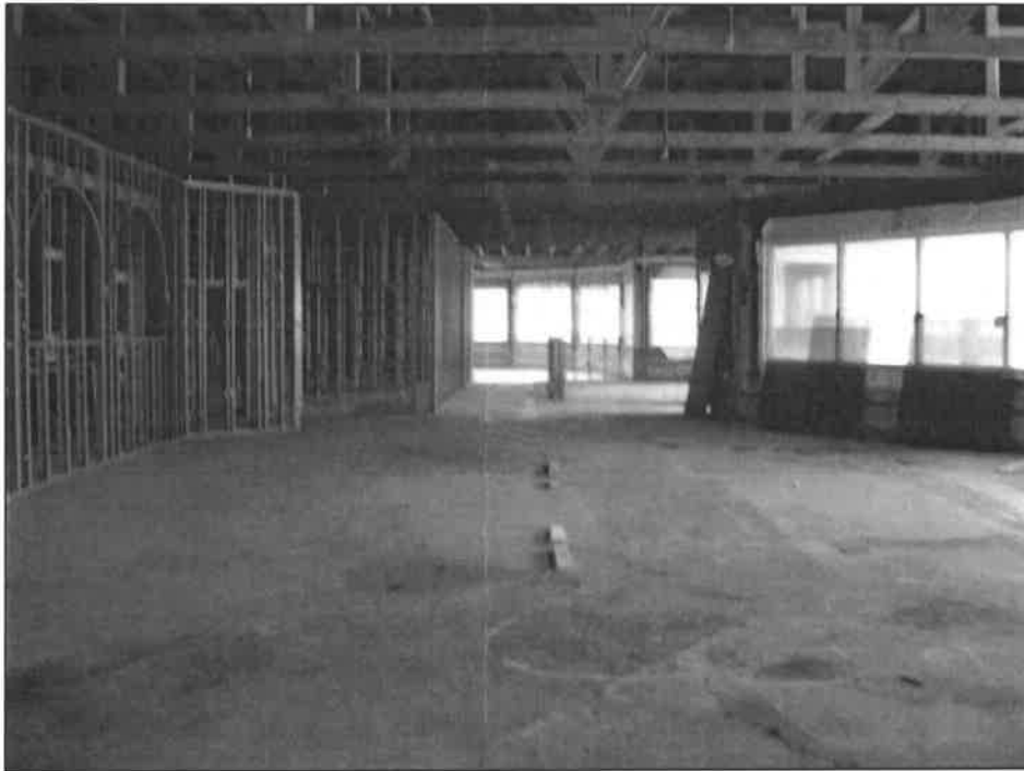
INTERIOR VIEW 2 ND FLOOR
