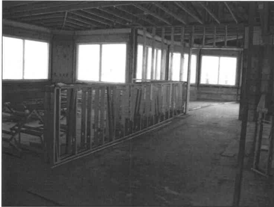
INTERIOR VIEW 2 ND FLOOR
