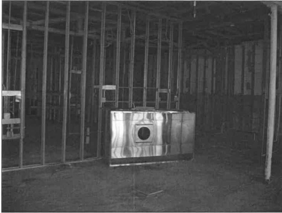
INTERIOR VIEW 2 ND FLOOR
