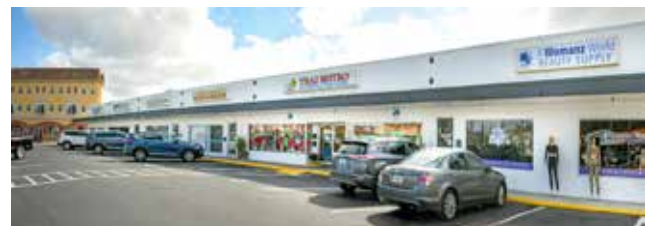
River Road Plaza existing conditions.
