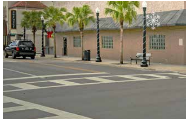
Existing condition along Grand Boulevard.
