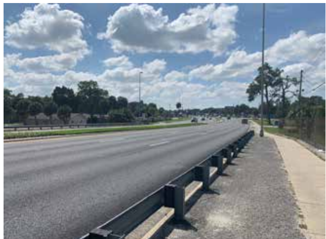
North Gateway from the Highway 19 Bridge.
