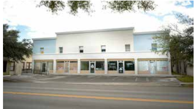
5840-5848 Main Street current conditions showing recent facade improvements.
