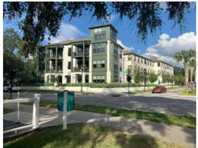
The Central represents a good example of how new development can engage and activate the park edges.
