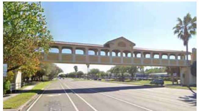
Example of a highway overpass from Lake Mary, Florida.
