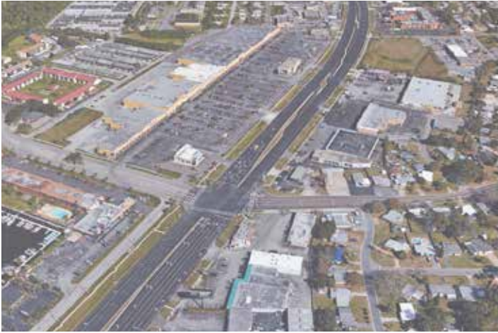
South Gateway existing conditions.
