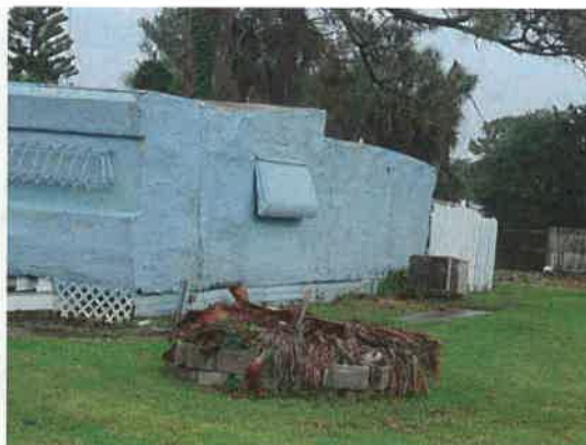
West side of home
