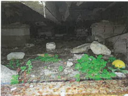
Block and piers foundation
