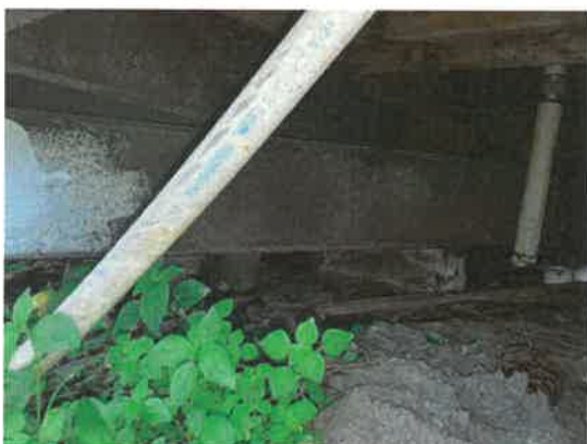
Additional view of block and piers
