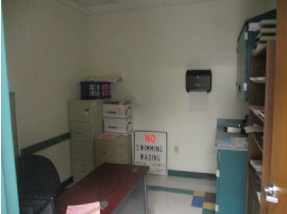
INTERIOR, FIRST FLOOR EXAM ROOM (USED AS OFFICE)
