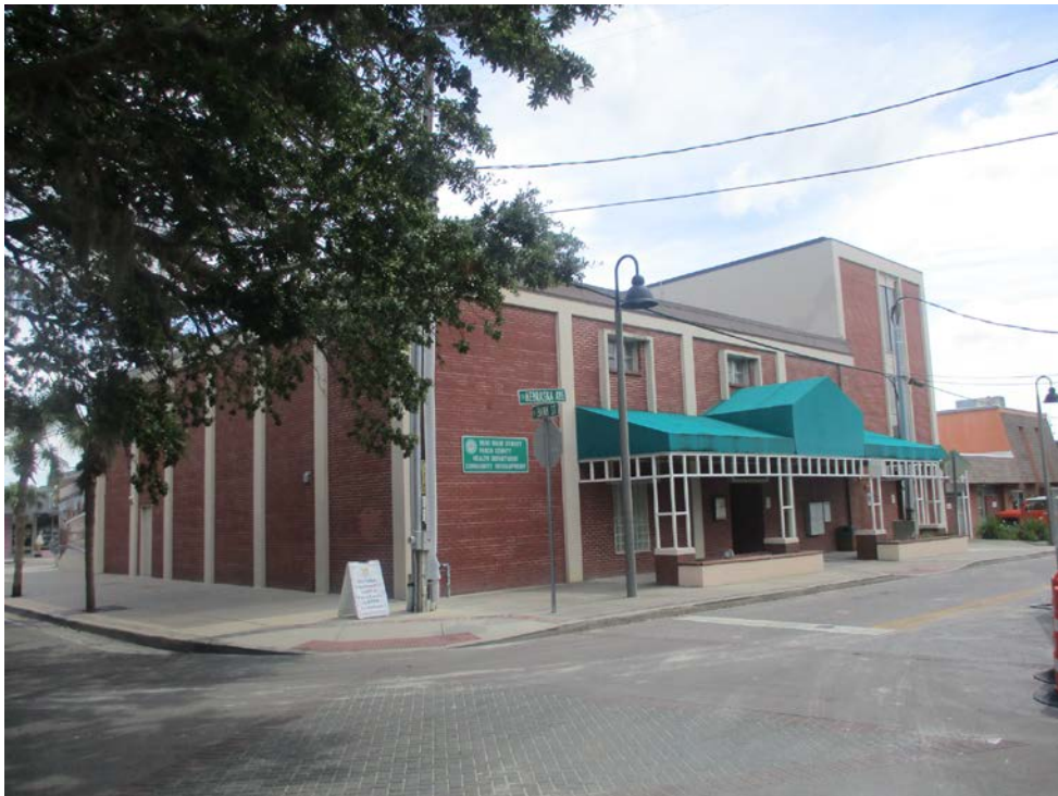
REAR AND WESTERN ELEVATIONS, FACING NORTHEAST
