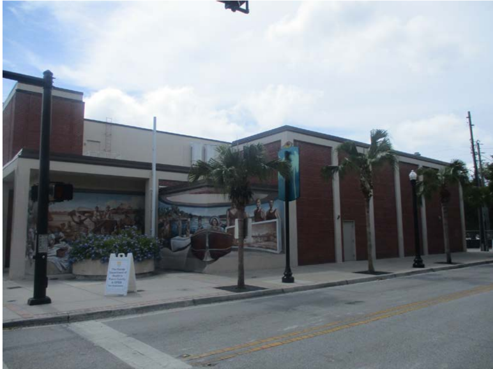
WESTERN ELEVATION FACING SOUTHEAST
