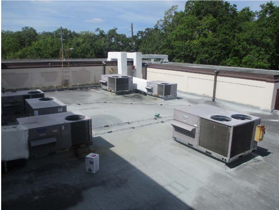
VIEW OF SUBJECT ROOF
