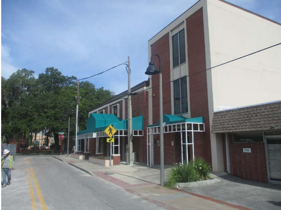
REAR VIEW OF BUILDING FACING NORTHWEST
