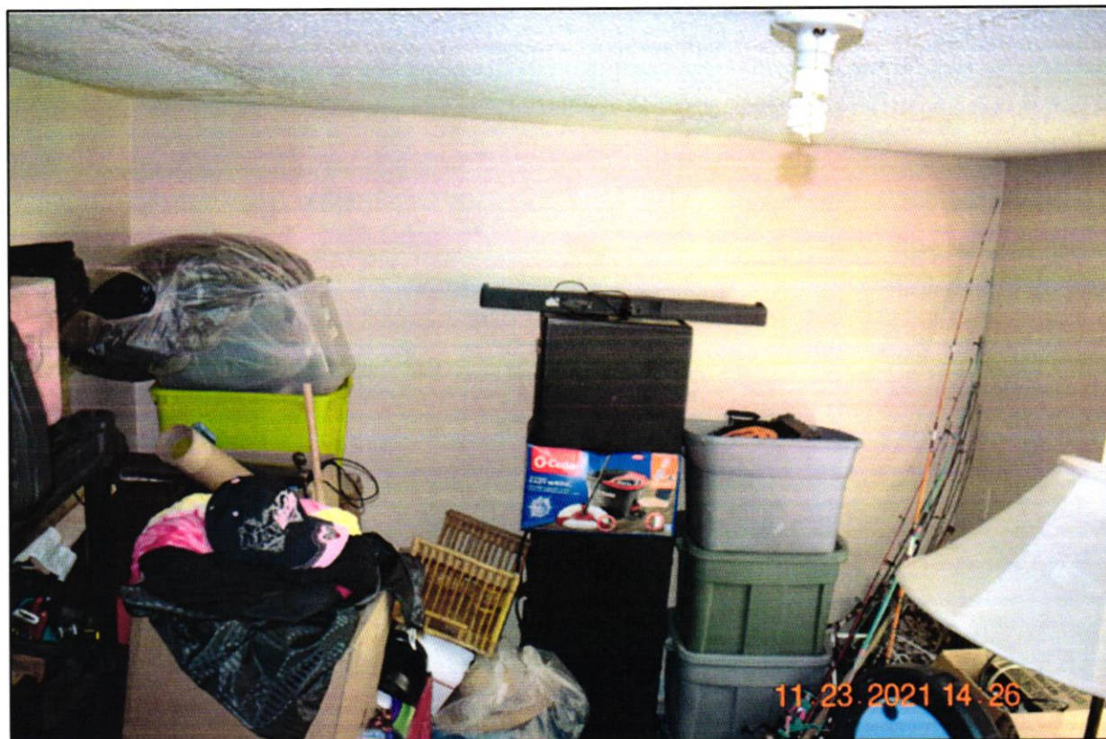
Mobile Home - Diffusers Required on Light Fixtures – National Electrical Code 410.11
