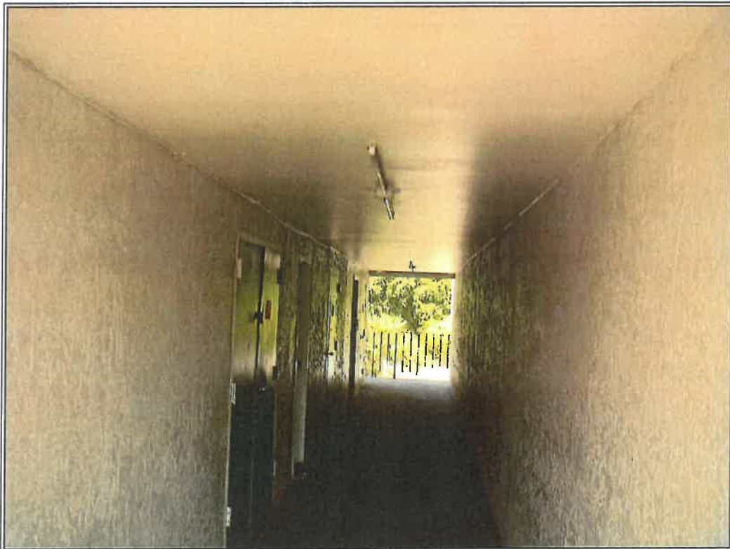
Interior Corridor for Service Areas
