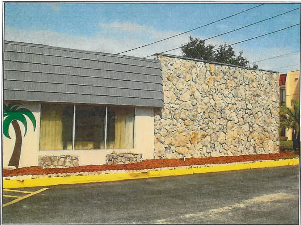
Exterior Detailing – Lobby Building
