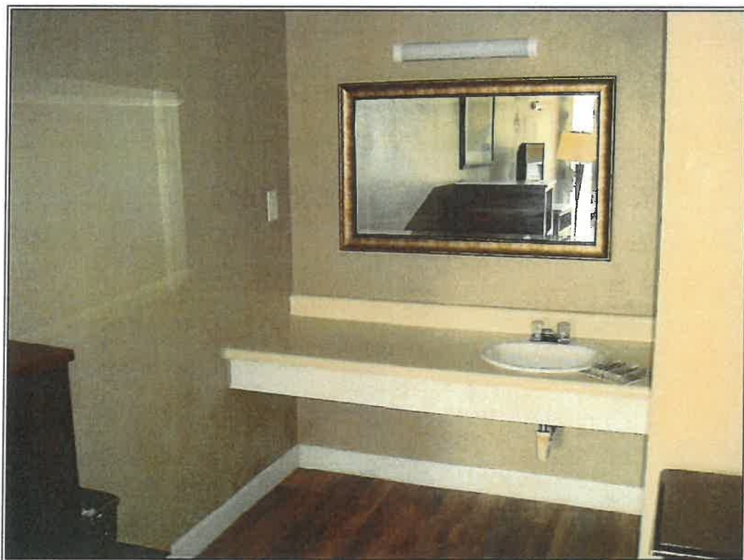
Sink and Counter Area
