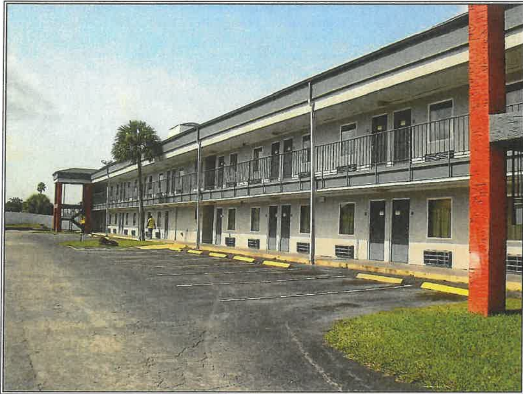
Front View of Hotel Building 1 (East)
