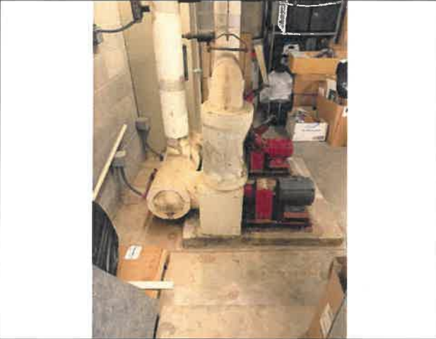
Photo 7 – Existing Chilled Water Piping
