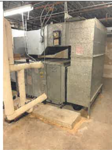
Photo 2 – Existing AHU-1
