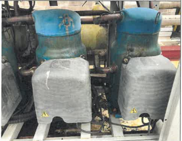
Photo 6 – Replaced Compressors
