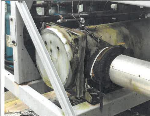
Photo 9 – Existing Chiller Insulation
