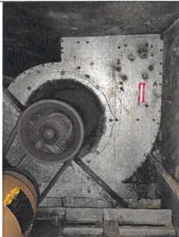
Photo 5 – Supply Fan Condition
