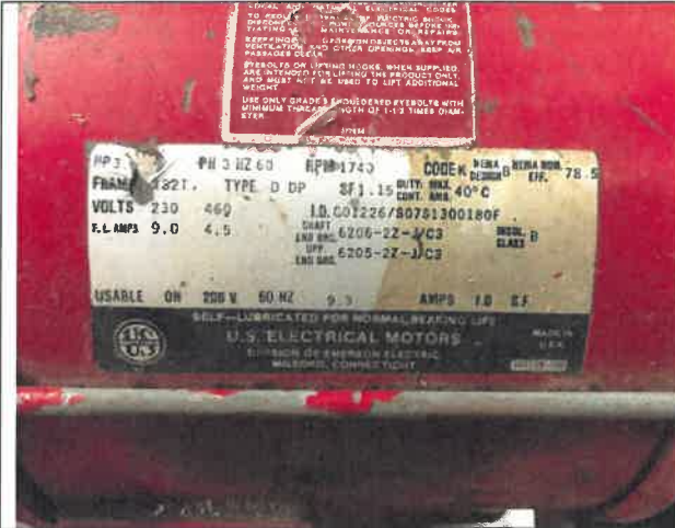
Photo 5 – Pump Nameplate
