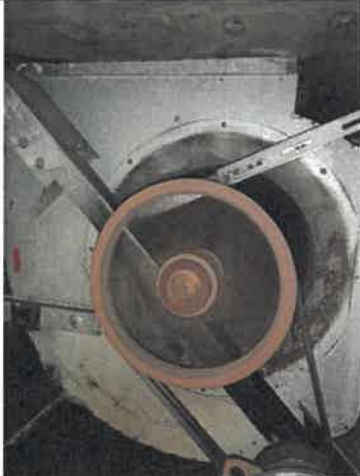
Photo 5 – Supply Fan Condition
