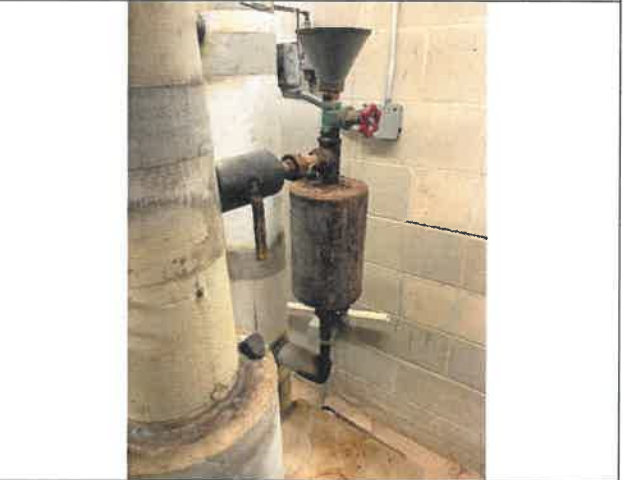
Photo 8 – Existing Chilled Water Component
