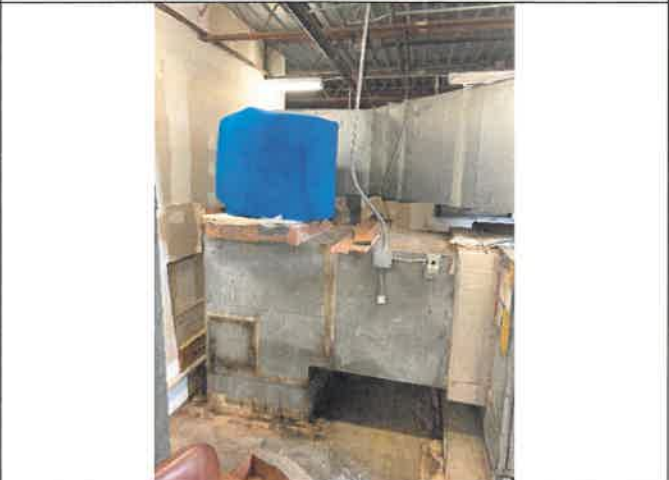
Photo 8 – Supply Ductwork
