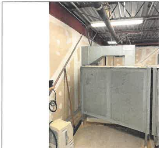
Photo 1 – Existing AHU-2
