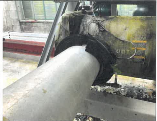
Photo 10 – Existing Chiller Insulation
