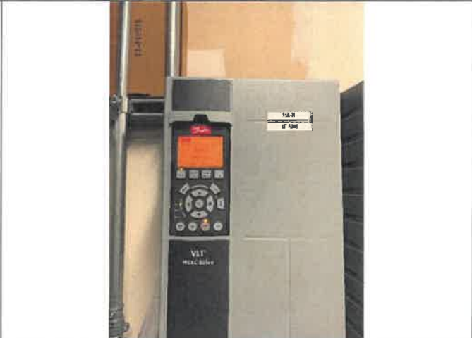
Photo 4 – AHU-1 VFD
