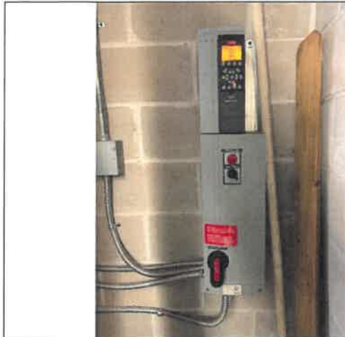
Photo 3 – AHU-3 VFD
