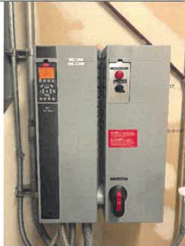
Photo 4 – AHU-2 VFD
