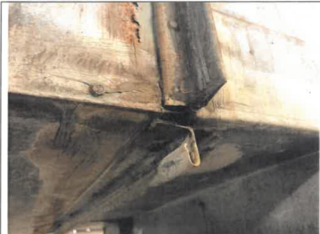
Photo 9 – Leaking Ductwork Seams
