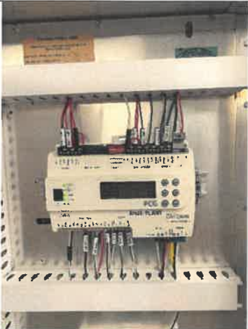
Photo 6 – AHU-3 Controls
