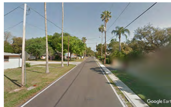
North River Road at Kentucky 20'
