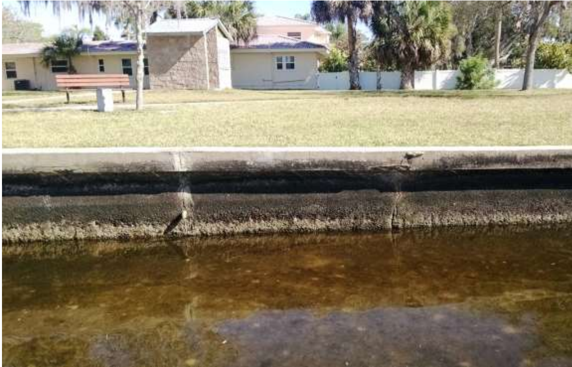
Figure 5 – Vertical Wall Crack
