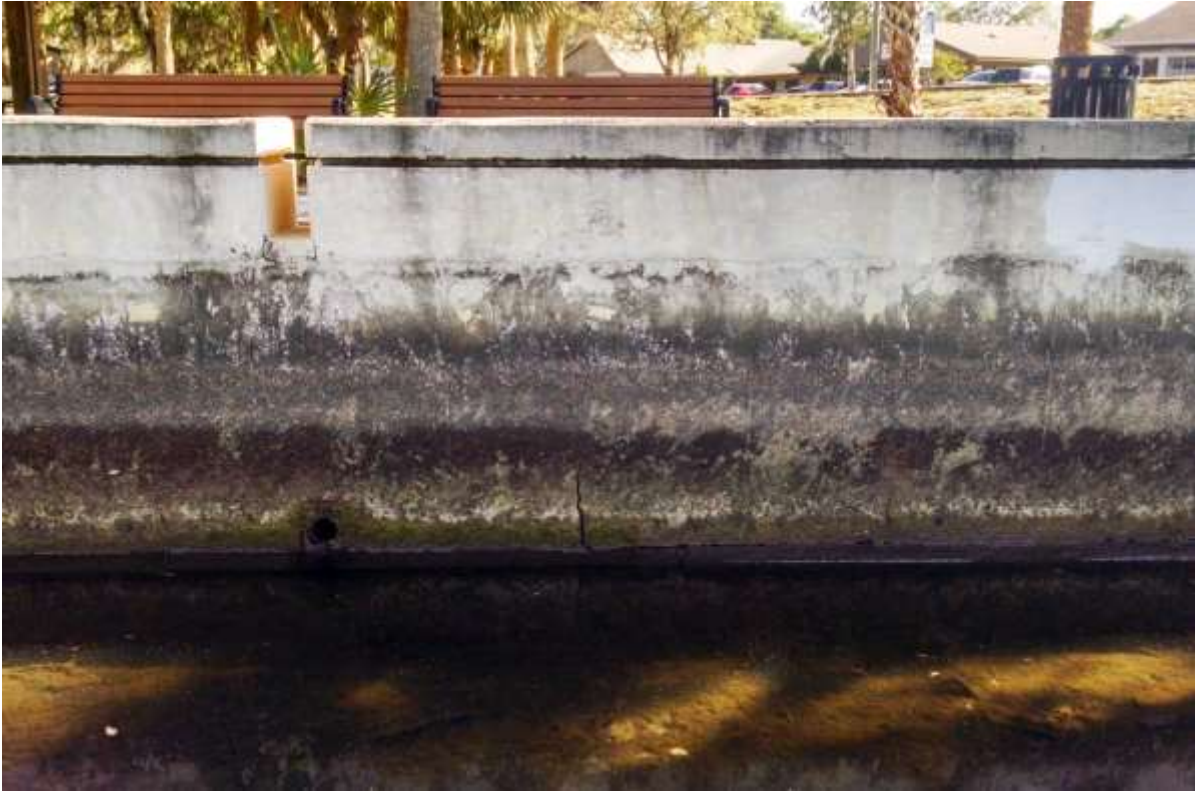
Figure 3 – Wall Crack at Base/Waterline
