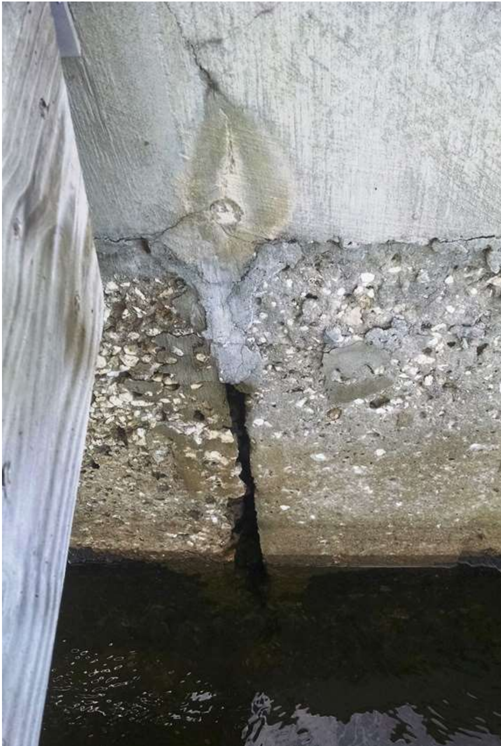
Figure 20 – Wall Joint Separation/Spalling
