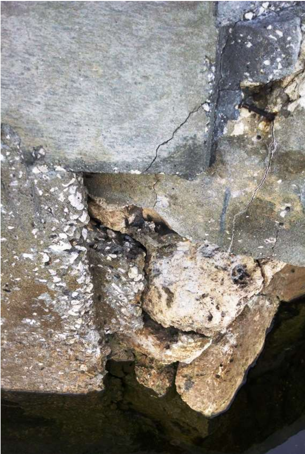
Figure 12 – Wall Crack/Spalling
