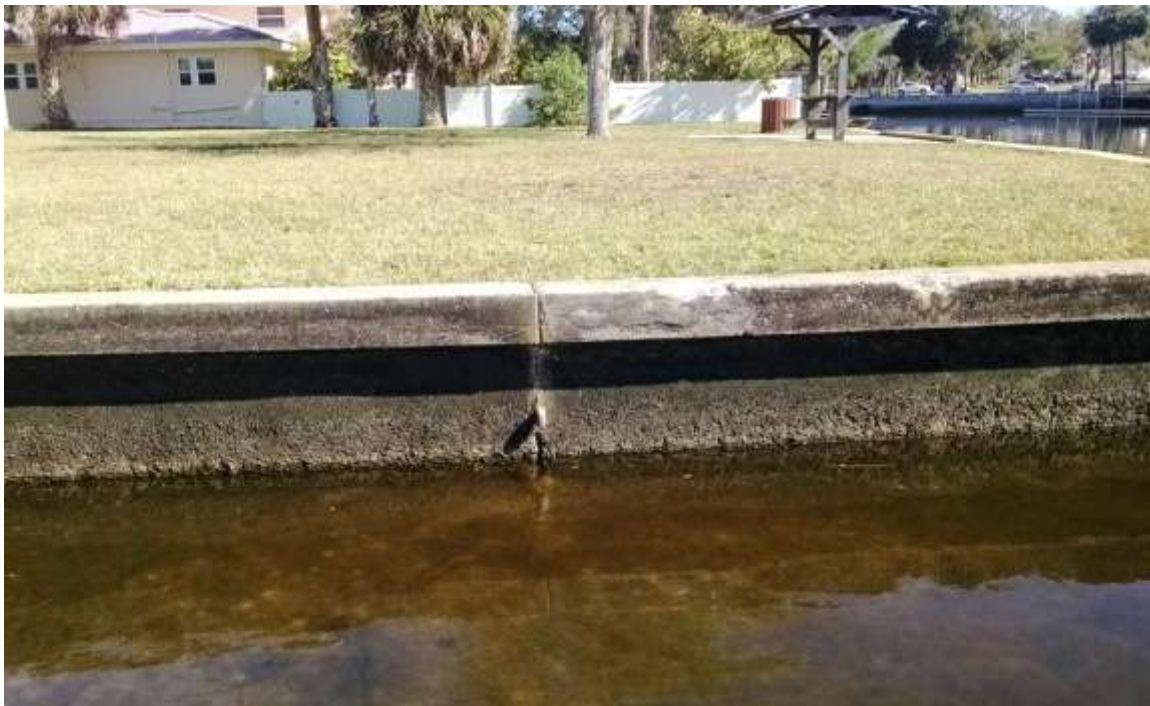
Figure 6 - Drainage Pipe at Wall Joint
