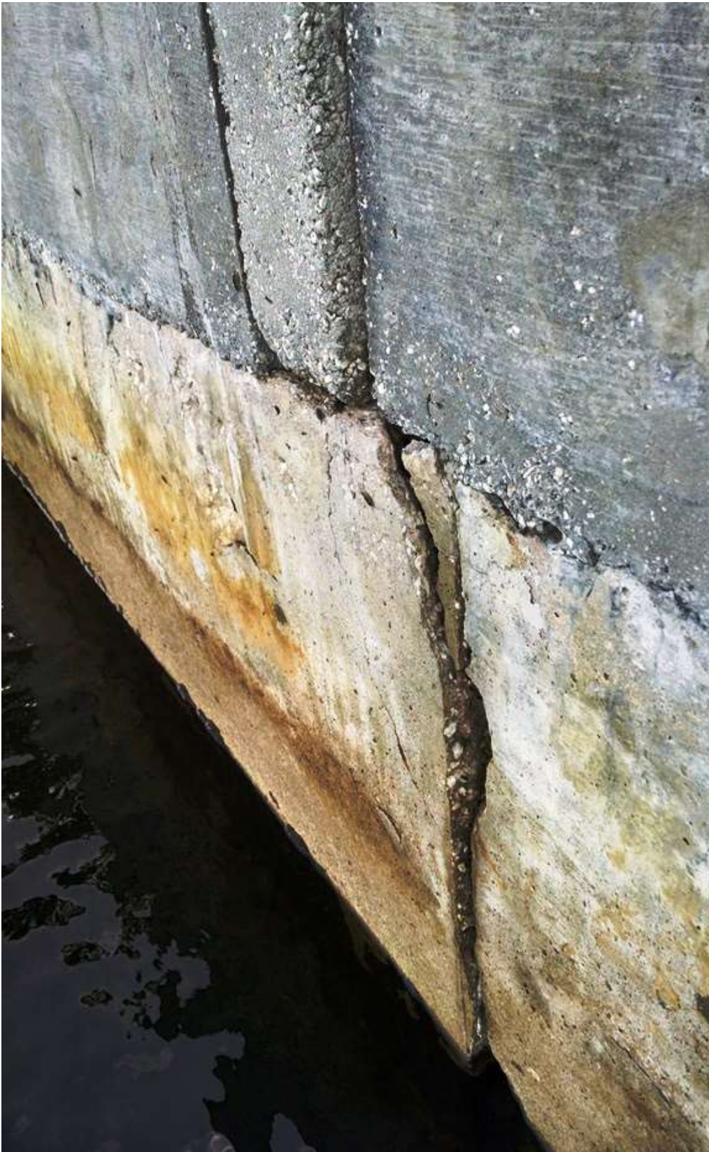
Figure 13 – Wall Crack/Shifting Outward
