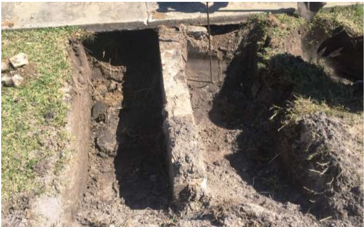
Figure 26 - Jasmine Park Bulkhead Concrete Tie-Back Excavation
