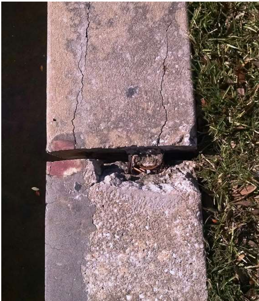
Figure 8 - Deterioration at Wall Joint
