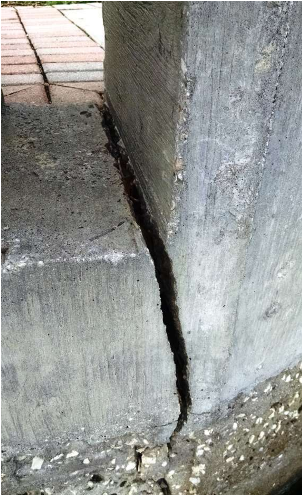
Figure 19 – Wall Crack at Spillway
