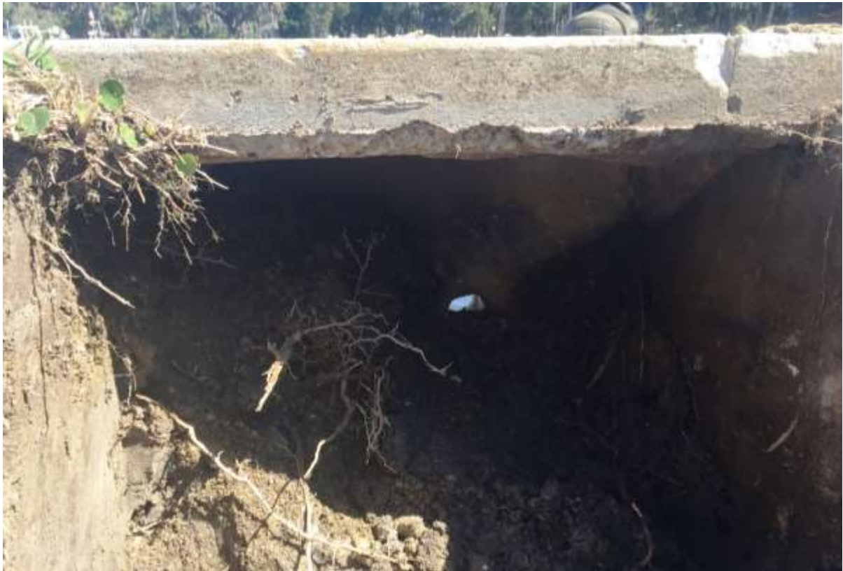
Figure 25 - Jasmine Park Seawall Drainage Hole Excavation – No Filter or Slotted Pipe Protection to Prevent Soil Erosion Through Hole
