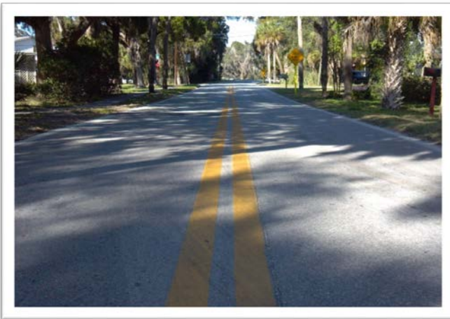
Figure 1 - Typical Roadway Grade 8 (Grand Blvd.)
