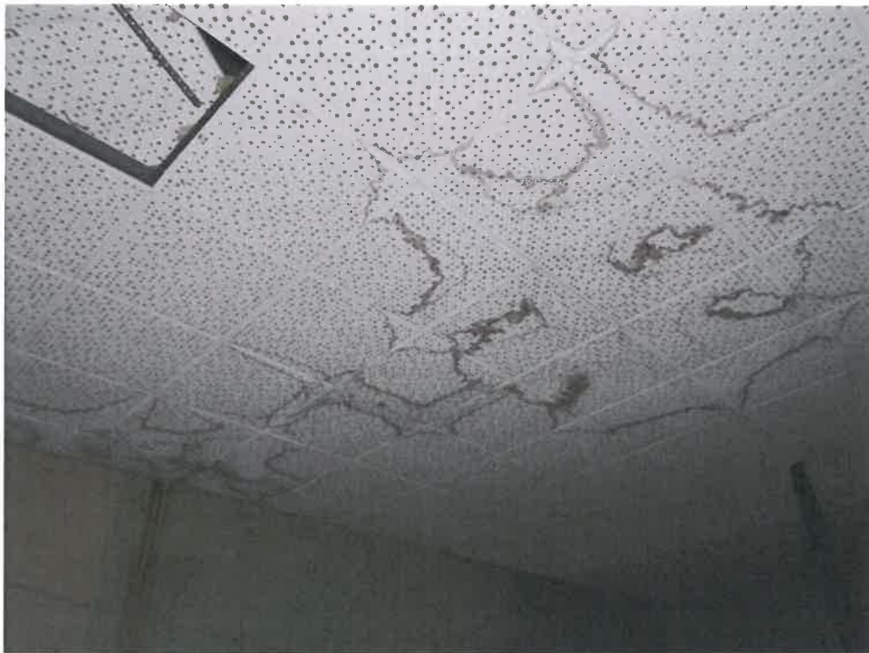
Figure 2: Stains on the original ceiling are visible in a hallway under the north section of roof.
