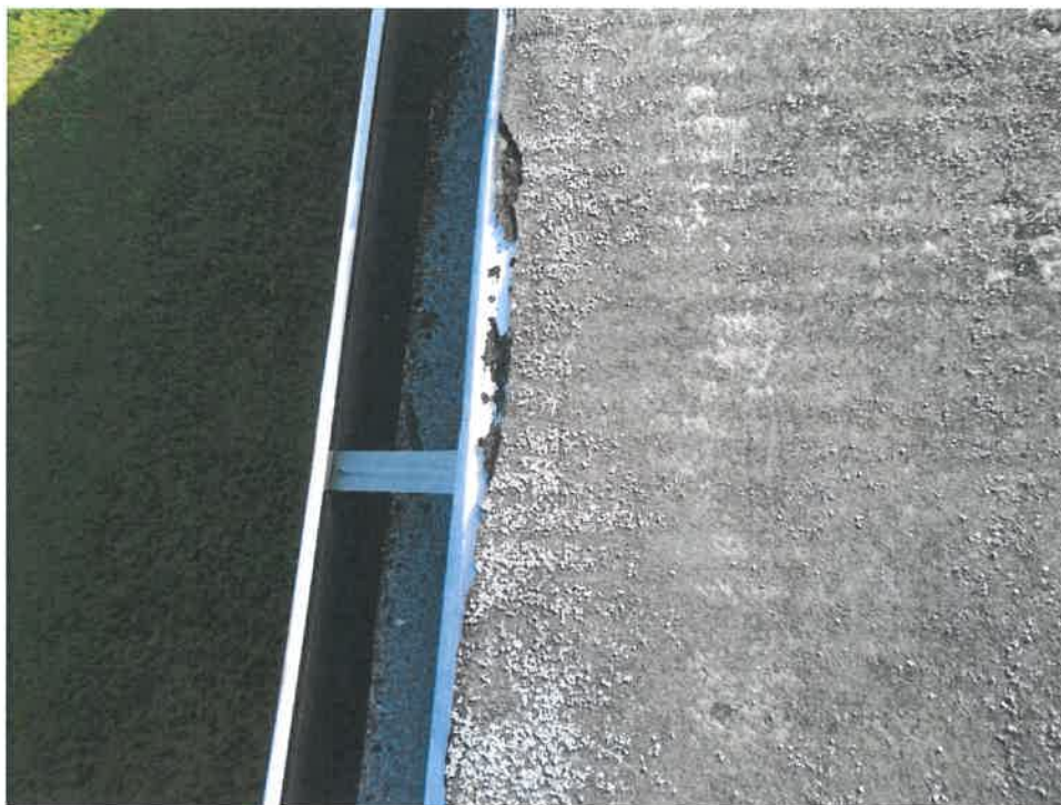
Figure 9: Torn and deteriorated membrane reveals portion of the drip edge around the perimeter of the roof.
