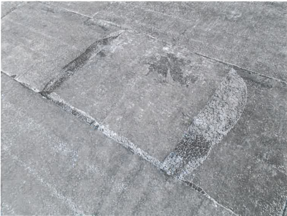
Figure 6: Extensive granule loss, deteriorated sealant, and patches are found on the north section of roof.
