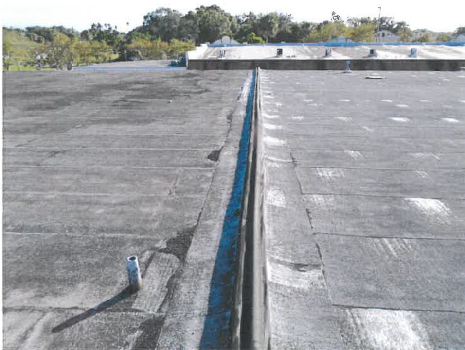
Figure 10: The expansion joint divides the north (left) section from the south (right) section of the roof.
