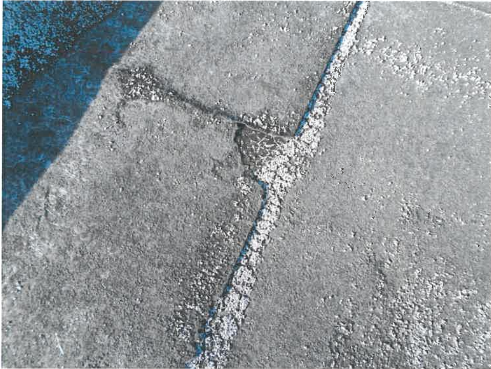
Figure 7: Deteriorated membrane and extensive granule loss are visible on the north section of roof.
