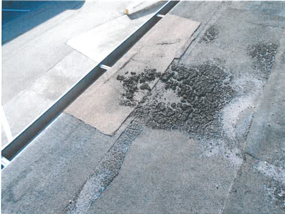
Figure 5: New patch, loose granules, and deteriorated sealant are found over the utility room where water was leaking from the ceiling.
