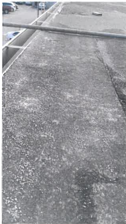
Figure 8: A small depression extends around the perimeter of the north section of roof.
