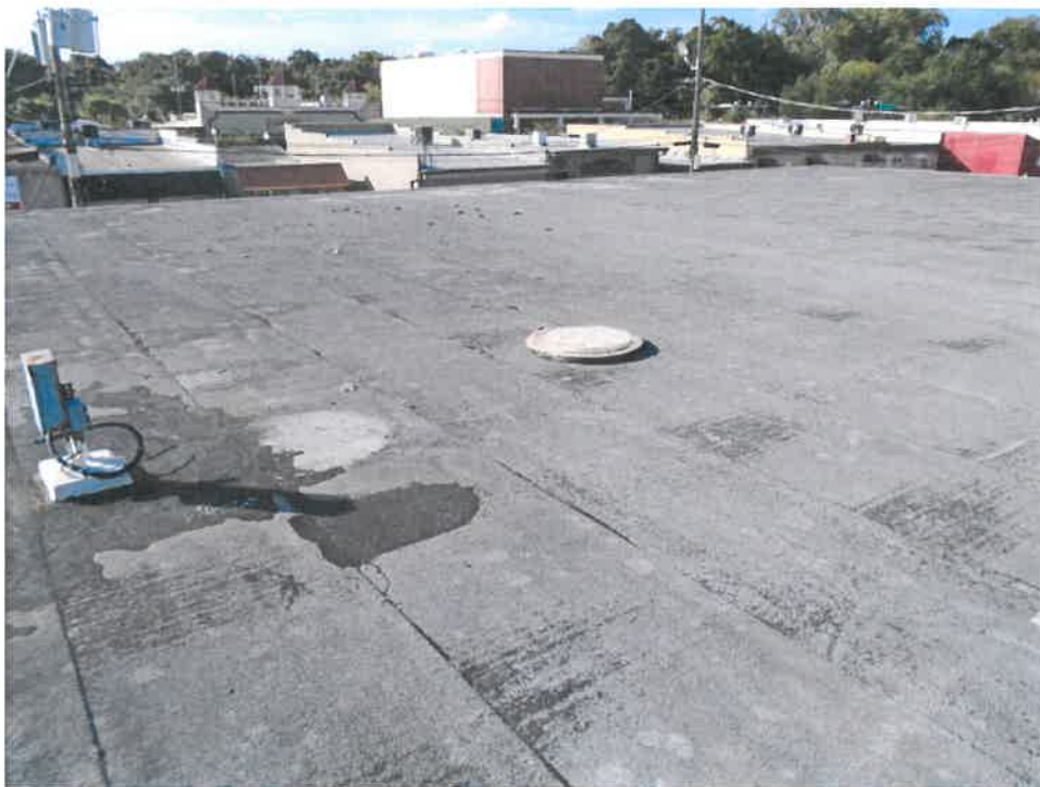
Figure 12: A concrete "disc", chunks of concrete, and sealant around an electrical utility box are visible on the south section of roof.
