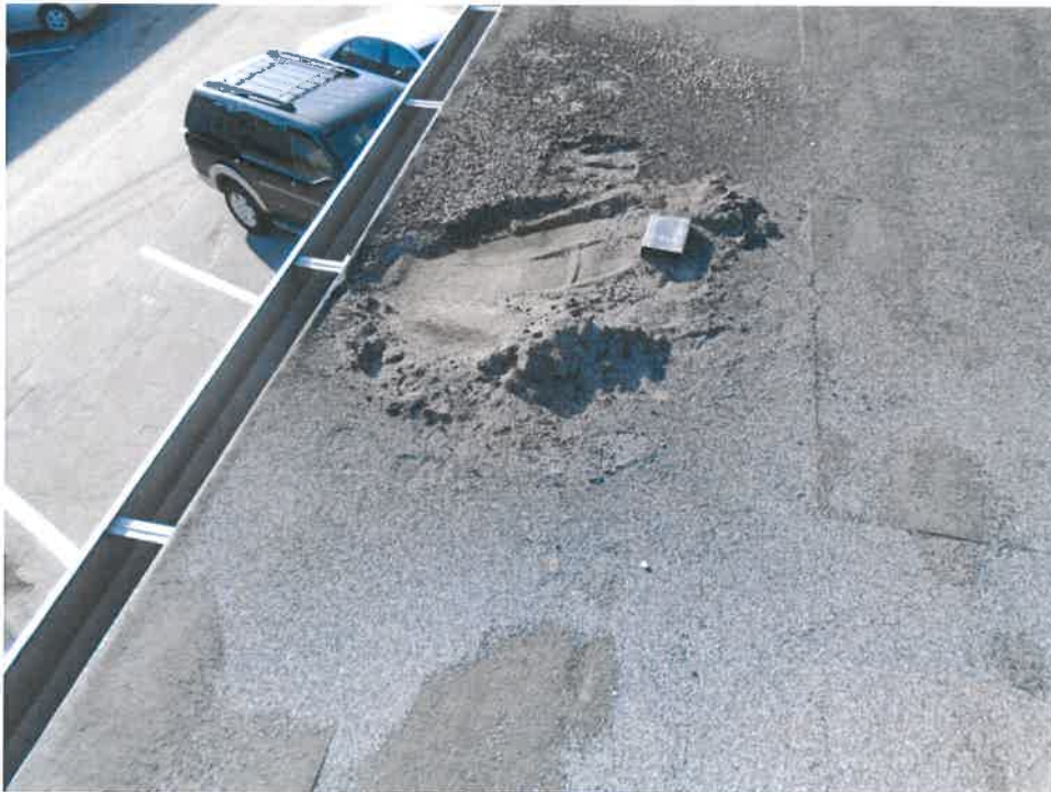
Figure 4: Depressed area in north section of roof where granules have accumulated over 1" thick.
