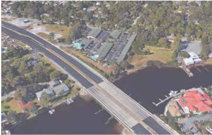
North Gateway existing conditions.
