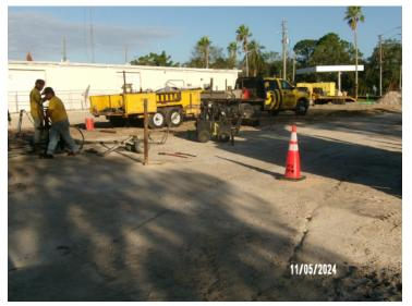
to prevent future soil raveling and downward migration of the soils into the underlying weathered limestone formation, fill existing voids within the overburden soils and improve the overall density of the soil profile and supporting soils beneath the building.
